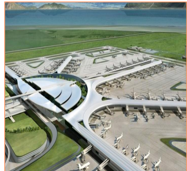
New Manila International Airport (Bulacan international Airport) – PHP735.6bn (US$13.3bn)
