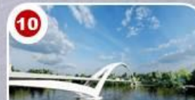
2nd San Juanico Bridge (4.85 km)
