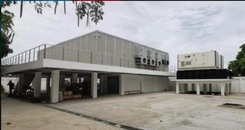
Luzon Bypass Infrastructure (LBI) Cable Landing Station, La Union
