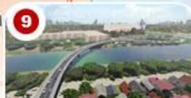
Marcos Highway - St. Mary Ave. Bridge
