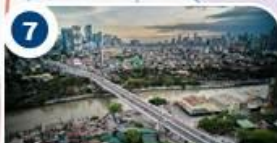
BGC-Ortigas Center Link Road Project
