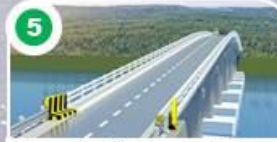
Tongsinah-Paniongan Bridge, Tawi-Tawi (0.57 km)
