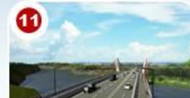
Kabayani St. - Matandang Balara Bridge
