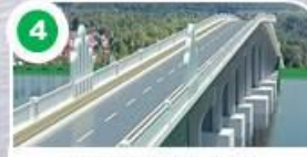
Nalil-Sikkat Bridge, Tawi-Tawi (0.54 km)
