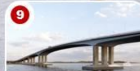
Cebu-Mactan Bridge (4th Bridge) and Coastal Road Construction Project (8.68 km)
