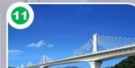
Panguil Bay Bridge (3.17 km)
