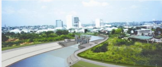
Pasig-Marikina River Channel Improvement Project, Phase IV
