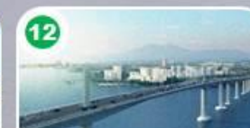
Samal Island-Davao City Connector Bridge (4.01 km)
