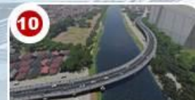
Homeowner's Drive - A. Bonifacio Bridge
