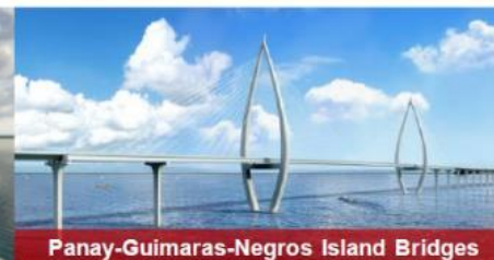
Panay-Guimaras-Negros Island Bridges
